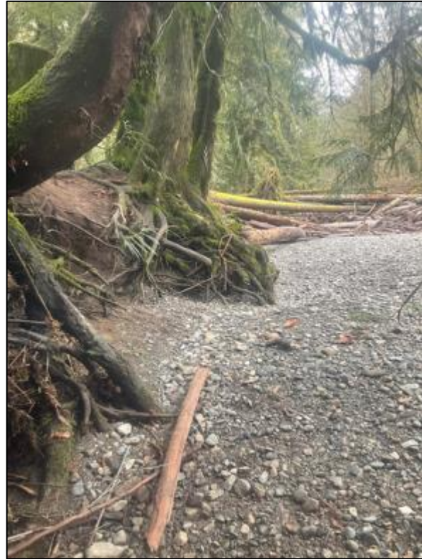
Figure 17. Winter storms are causing extreme erosion and bank instability along the Koksilah River.
