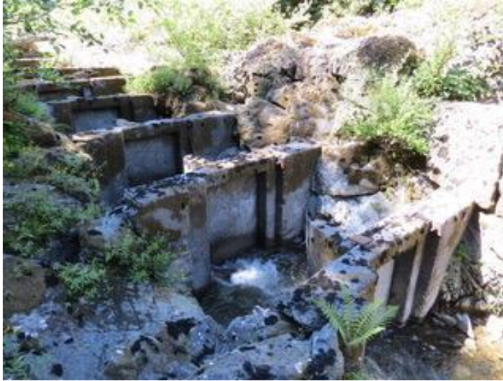
Figure 51. Fish way constructed to improve fish habitat.
